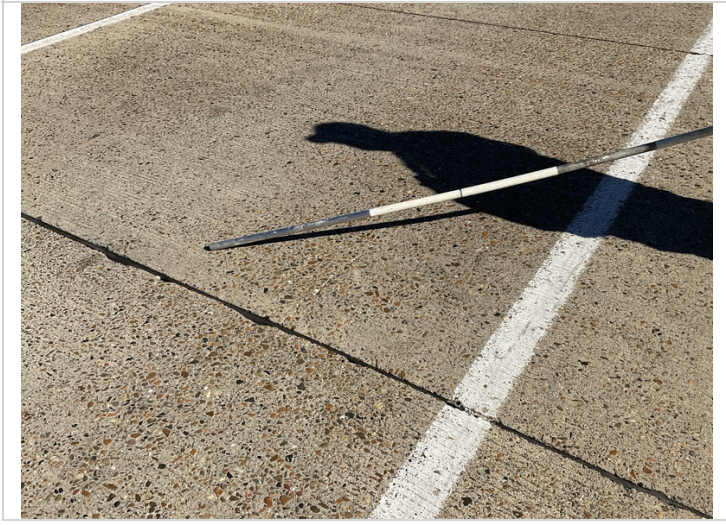
Span 2 longitudinal crack.
