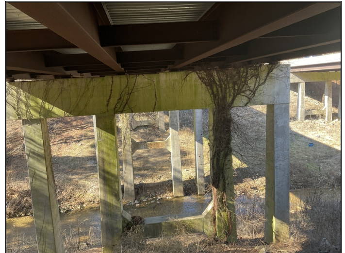
Vines growing on columns and cap at bent 4.
