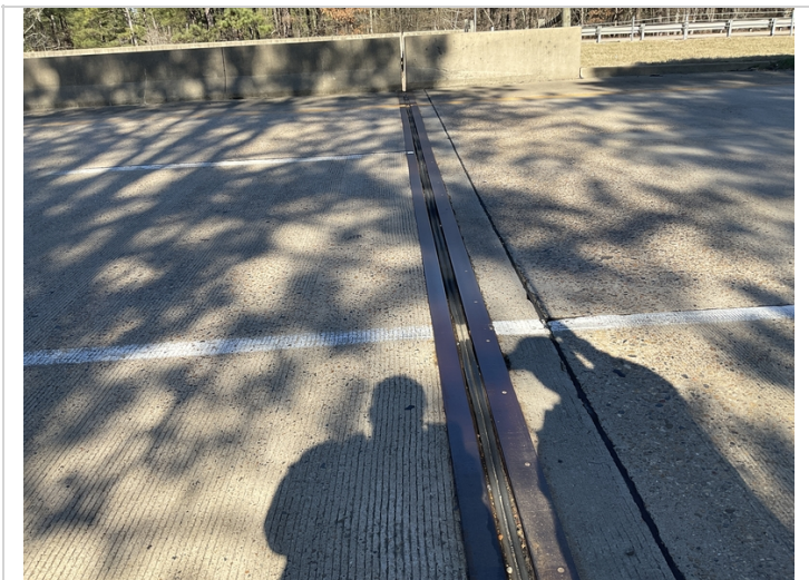
Bent 5 joint seal has lost bond.
