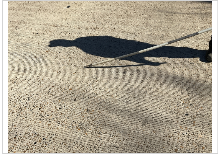
Span 4 longitudinal crack.
