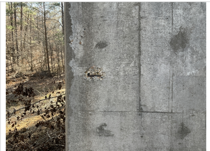
Bent 2 column 2 has small spall with exposed rebar on left.
