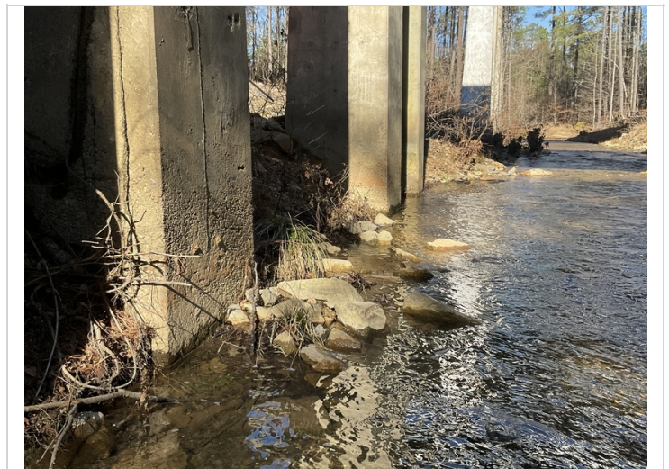
Bent 3 columns 2 & 3 have abrasion at waterline.
