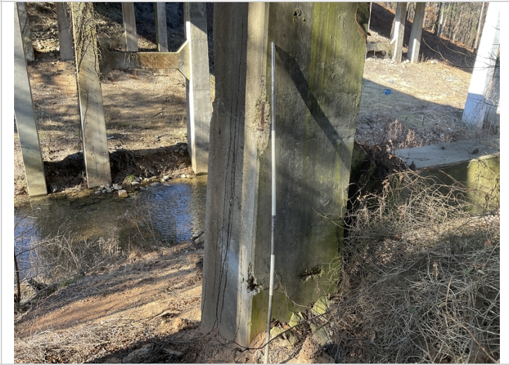
Bent 4 column 3 ahead side spalls with exposed rebar.
