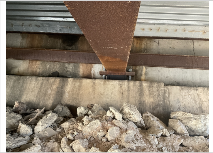
Bent 5 cracks with efflorescence in back wall.
