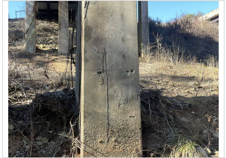
Small spalls with exposed rebar bent 3 column 3 ahead.
